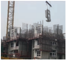
Lifting anchors are widely used at precast concrete that speeds up the construction progress
