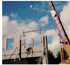
Remote Release Clutch System will eliminate needs to climb up at height
